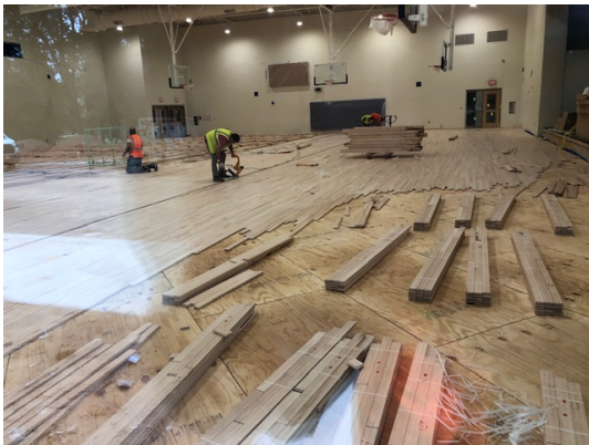
Gym floor install at WPA
