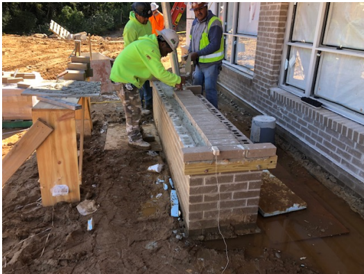
YMCA canopy brick topcaps installed
