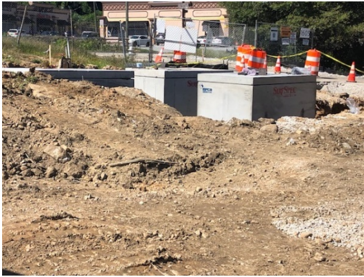
WPA water vaults installed
