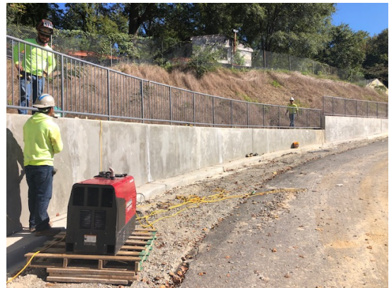
Retaining wall guardrail installed
